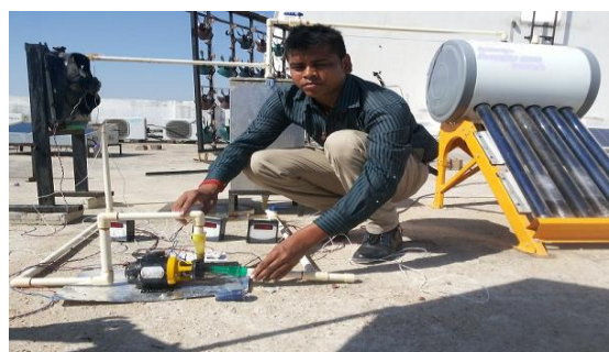
Fig.1. Connecting C P V C pipe and Tullu pump in a system
